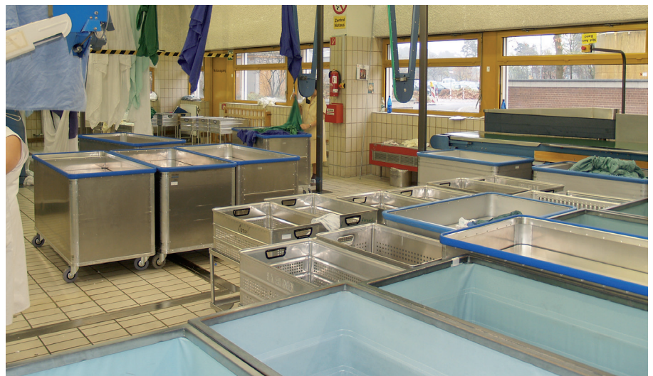
Spring-loaded base trolleys and baskets in a laundry
