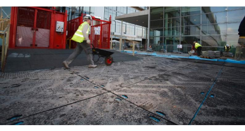
EuroMat<sup>®</sup> is a market leading medium duty ground protection mat designed as an ideal manhandle-able solution in a wide range of applications including temporary roadways, work pads, depot storage areas, or as pedestrian access. Thanks to its flexible design, the mat is able to follow the contours of undulating or sloping ground conditions.
