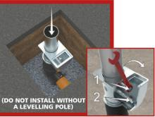
5 Surround with C30/37 minimum strength concrete. Vibrate to remove air.
