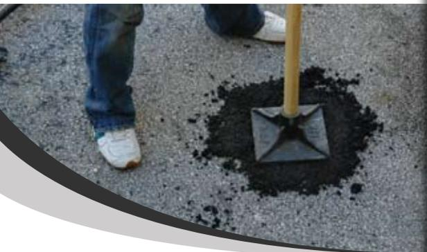
**C** Compact the EZ STREET Cold Asphalt to just over the level of the existing pavement.
