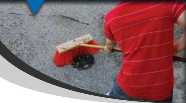
**A** Sweep out area to be patched. Make sure to remove all loose debris, broken pieces of pavement and dust.
