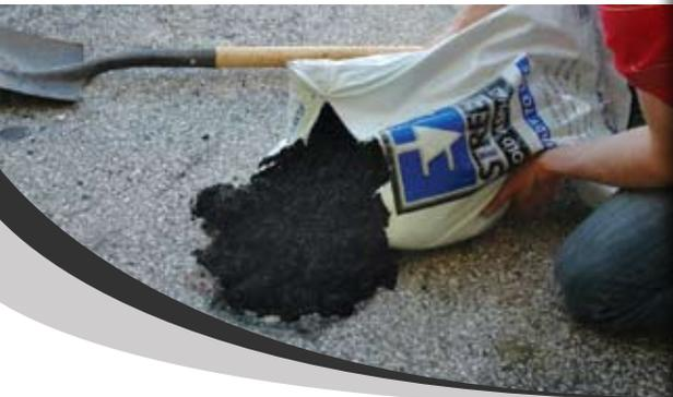
**B** Fill pothole with EZ STREET Cold Asphalt. For holes deeper than 50mm, compact material in 25mm - 50mm layers.
